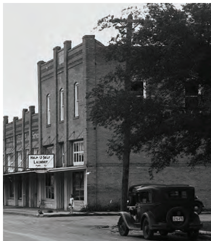
In 1934, the Woodmen Hall building housed a self-service laundry on the first floor
